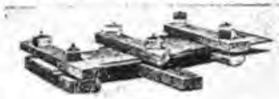
FIG. 6.—Clamps made of rough "two-by-fours" for straightening water-soaked table tops or leaves.
