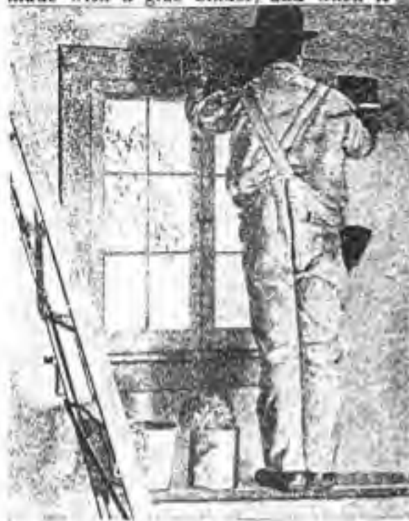
FIG. 30.—Kalsomine is blown on freely with a broad brush made especially for this purpose. Only one coat is necessary.
