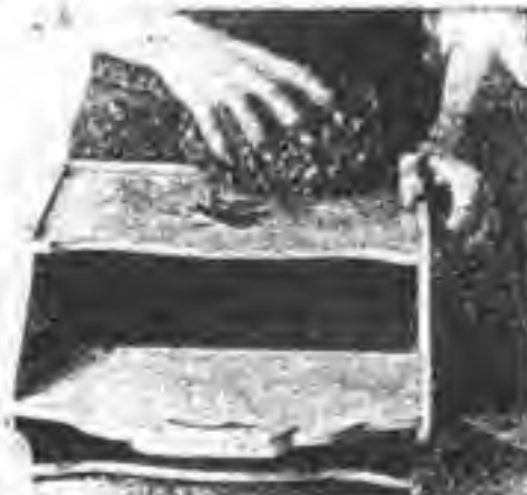
FIG. 18.—The surface is cleaned first with clear water, then with gasoline diluted with water.
