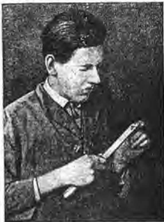
FIG. 3.—Thumb nail test for a chisel; if it "takes hold," it is really sharp.
