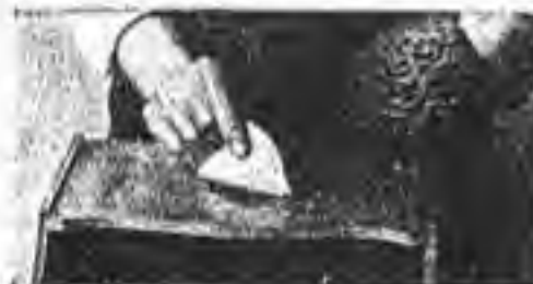
FIG. 17.—After being saturated with water, the paper backing is either lifted up or slipped off.
