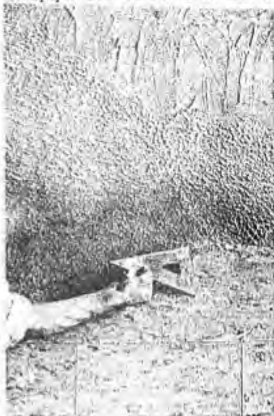
FIG. 31.—Developing a travertine finish. Greenspar is blown on the joint after it has been stippled.
