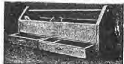
FIG. 36.—This extremely compact and convenient portable tool box has divisions for saws and planes; also two drawers for chisels and small tools.
