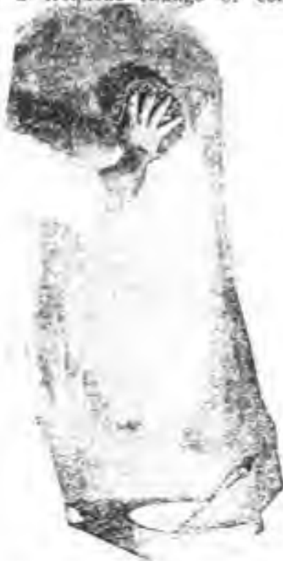
FIG. 37.—Old kalsomine must be washed off before new is applied.
