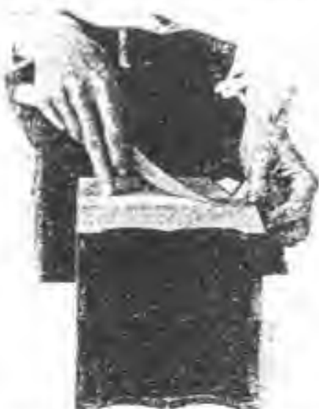
FIG. 6.—After it has protected one part while another is being painted, the masking tape is peeled off.
