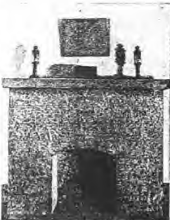
FIG. 33.—A fireplace of wood, wall board, and plastic paint. The small chest on the mantel and the decorative part above were stenciled with plastic paint.
