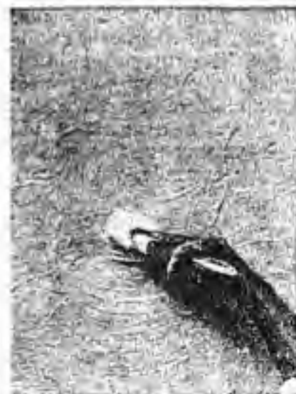
FIG. 28.—Semicyclic sweeps of a 4-in. wall brush produce the so-called "monastic" texture.
