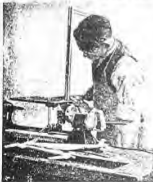
FIG. 28.—The grooves for the head and bottom pieces are cut after the frame is assembled and dried.
