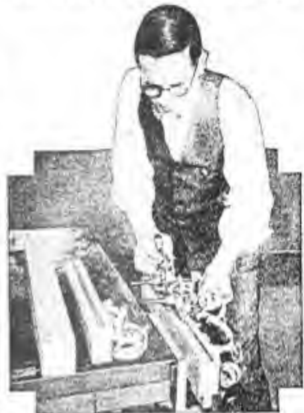
FIG. 13.—Using a combination plane to plow grooves in the rails, strips can be nailed on instead of making grooves.
